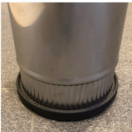
Flue seated correctly.
