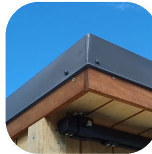
REAR FASCIA BUTT IN TO SIDE FASCIA
