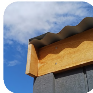
REAR FASCIA BUTT IN TO SIDE FASCIA
