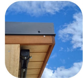
REAR FASCIA BUTT IN TO SIDE FASCIA
