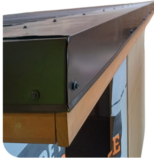
SIDE BARGES SCREWED OFF AT 600MM CENTRES
