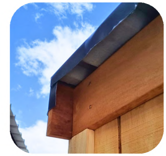
REAR FASCIA BUTT IN TO SIDE FASCIA
