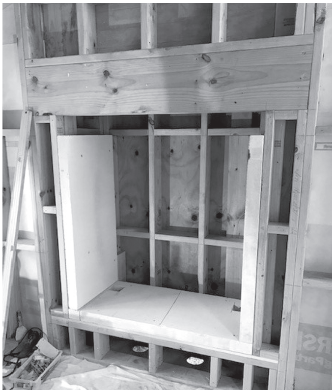
Timber Frame-out with AAC block panels and air vents
