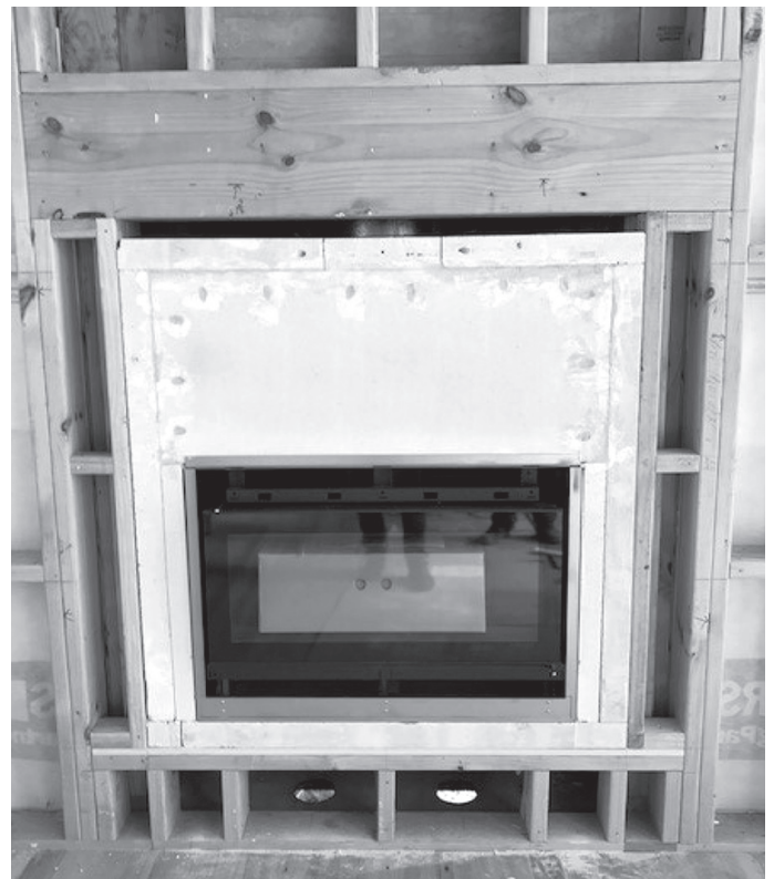
Timber Frame-out with AAC block panels and air vents
