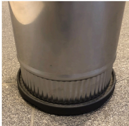
Flue seated correctly.
