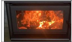
**STEP 5** – When the paper, kindling and the medium logs are well alight, shut the door completely.
